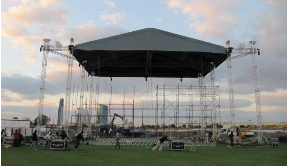
Photo: Showtech, Dubai. Build of a ST Roof.
